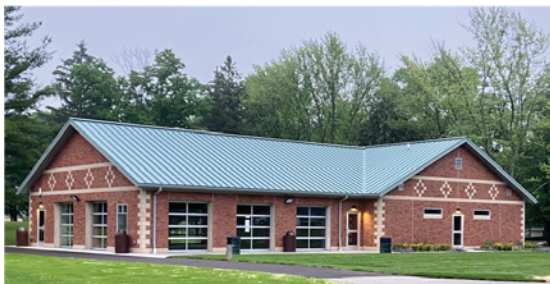
Firemen's Park Indoor Pavilion W162N11862 Park Avenue
